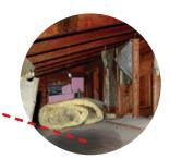
Leakage in attic after driving rain Possible causes: Degraded or inadequate shingle underlayment; deteriorated flashing
