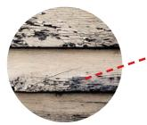
Blistering and/or peeling of outside paint Possible cause: Excessive moisture or high humidity due to poor attic ventilation
