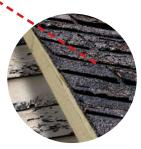
Roof shingle, sheathing, and siding decay Possible cause: Poor attic ventilation
